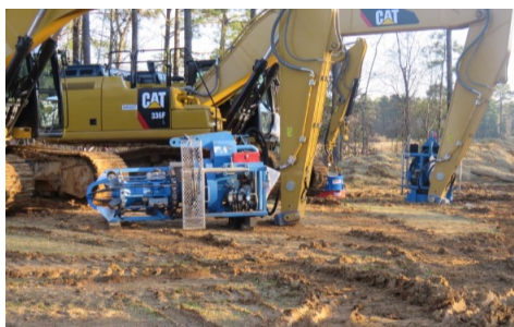
ACP pipeline construction near Pleasant Hill
