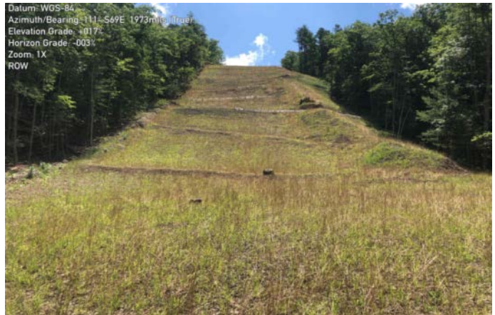
Spread 3A – Stabilized ROW
