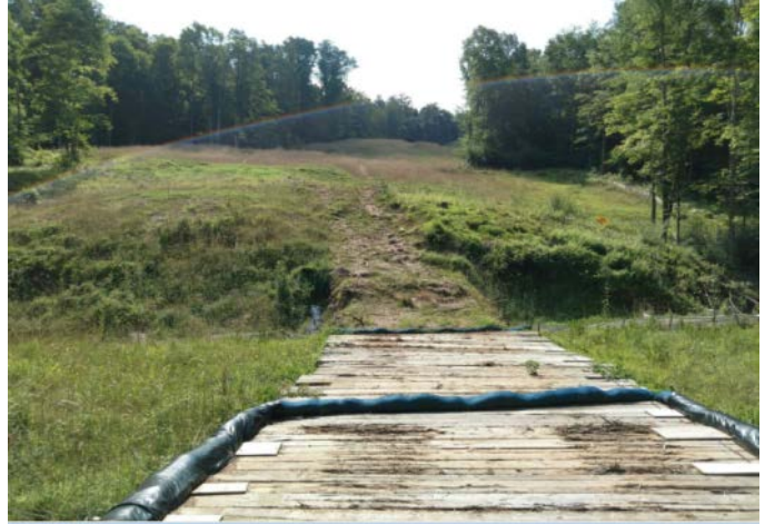
Spread 1-2 – Stabilized ROW
