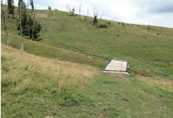
Spread 1-1 – Stabilized ROW
