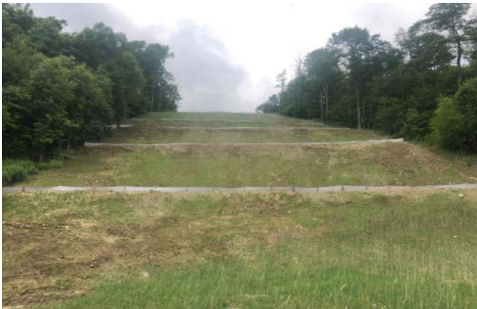
Spread 2A – Stabilized ROW / ECD inspection
