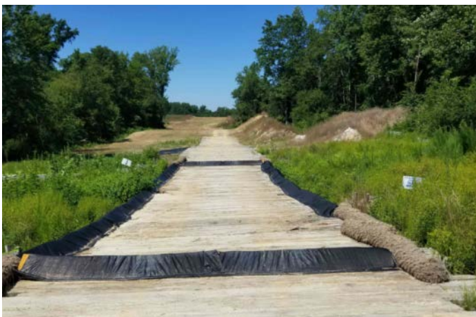
Spread 8 – Stabilized ROW
