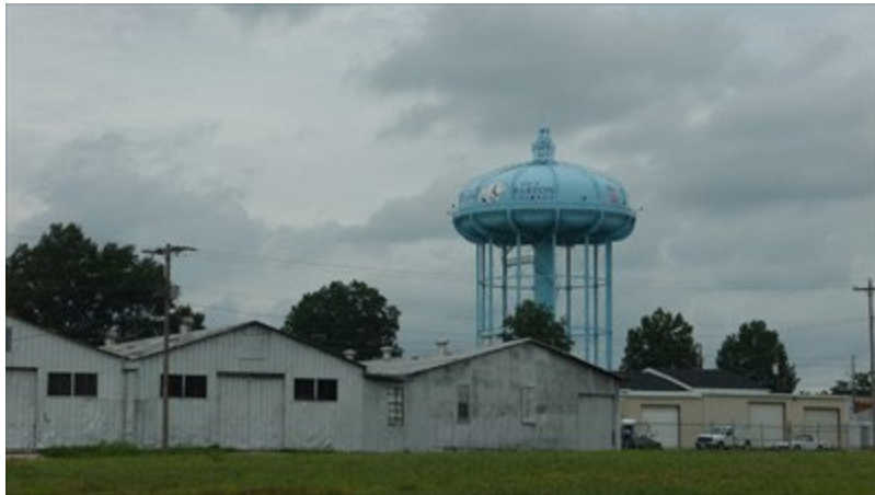
Wilson, North Carolina Water Tower. Source: Waymaker
