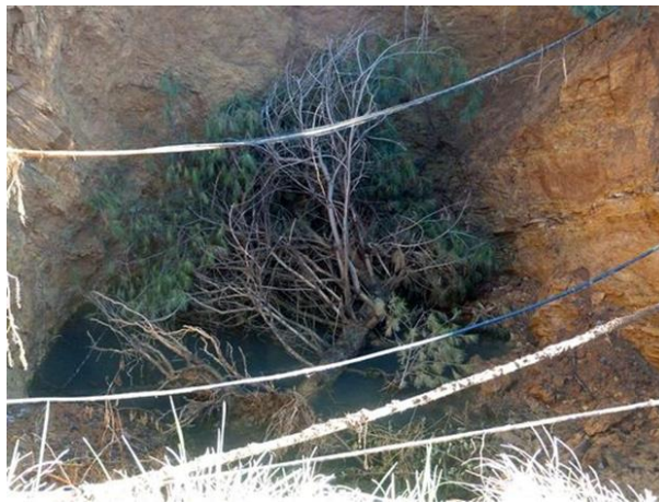
Thirty foot-wide sinkhole, with exposed cable lines ( http://www.newsleader.com/story/news/local/2015/11/14/sinkhole-sparks-safety-pipeline-concerns/75768270/ ).
